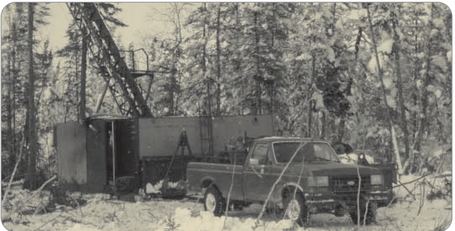
DRILLING BELOW PREVIOUS MINE WORKINGS AT JASPER
